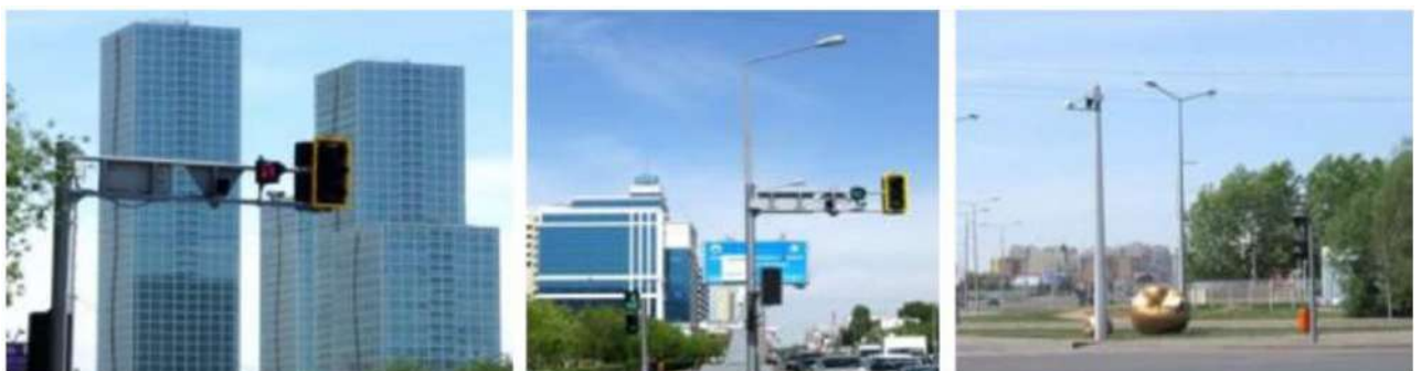
Figure 4 – Traffic lights in Kazakhstan
